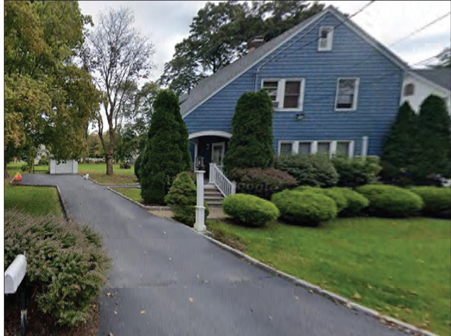
FRONT VIEW OF EXISTING HOUSE - LOT B
